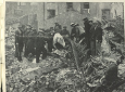
A PART OF THE HEAVILY DAMAGED BUILDING. THE BUILDING WAS HEAVILY DAMAGED BY THE GERMANS.
