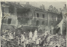
A PART OF THE HEAVILY DAMAGED BUILDING. THE BUILDING WAS HEAVILY DAMAGED BY THE GERMANS.
