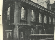
A PART OF THE HEAVILY DAMAGED BUILDING. THE BUILDING WAS HEAVILY DAMAGED BY THE GERMANS.
