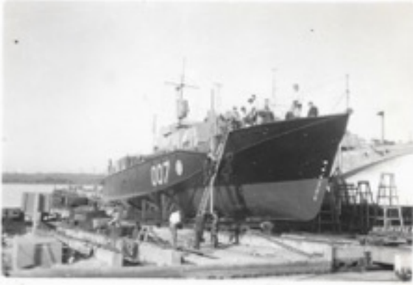
LRRC 007 July 1945 Underwater Inspection at Poole
